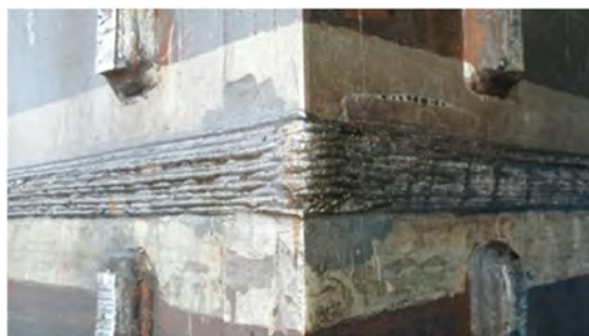
写真-14 溶接外観
