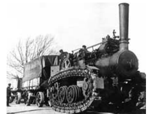
写真—15 Full Track-Laying
