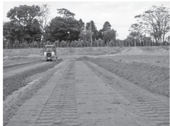
図-6 3D-MC<sup>2</sup>の整地性確認状況
