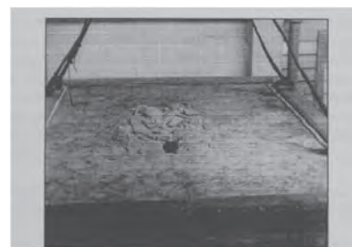
d) Explosive spalling
