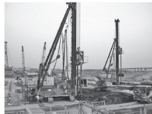
写真-8 地盤改良工 (SDM-Dy)
