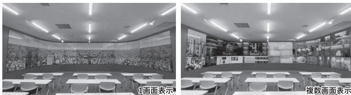
図-2 Smart Control Center (SCC) (3行×12列:平面24枚, 曲面6枚)
