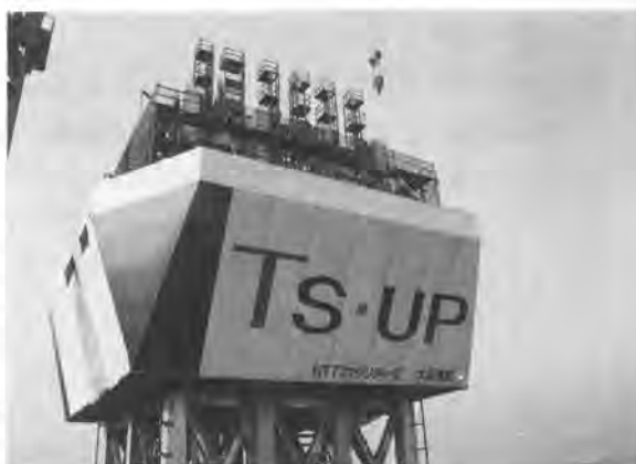
写真-1 Ts-Up 工法外観
