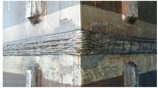
写真-14 溶接外観
