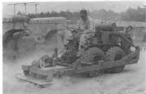
写真-4 平板振動締め固め板装着
