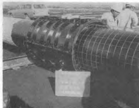
写真-2 溶接金網、型枠
