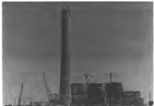
写真-1 Boiler & T/G Building
