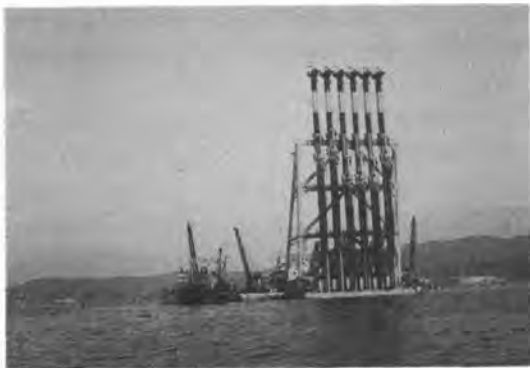
写真-2 砂杭打船 (6連装)
