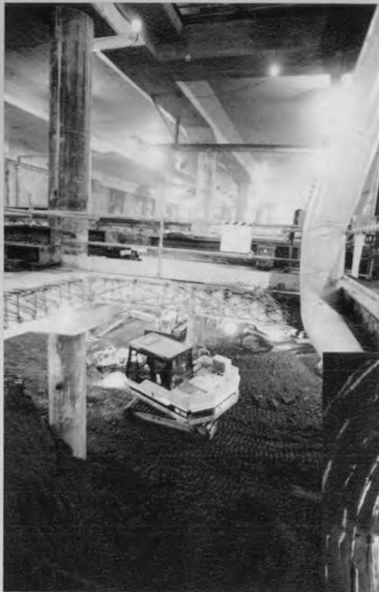
⇨ B3階の掘削
