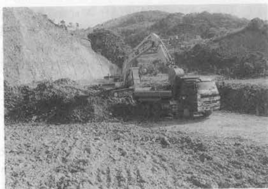
写真-6 10t車の積込
