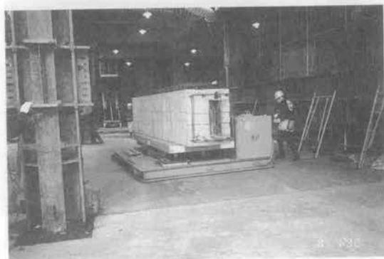
写真-56 空気浮上式PC梁運搬取付機ATB (Air Transporter Builder)
