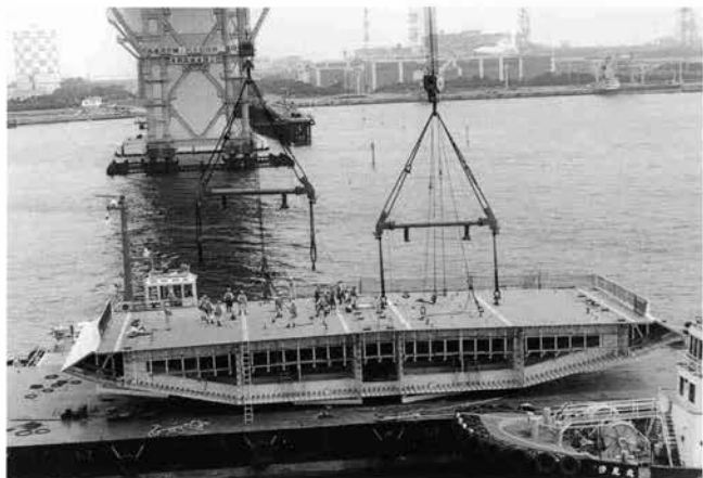
桁吊具装着
