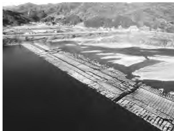
写真-1 着工前南岸堰
