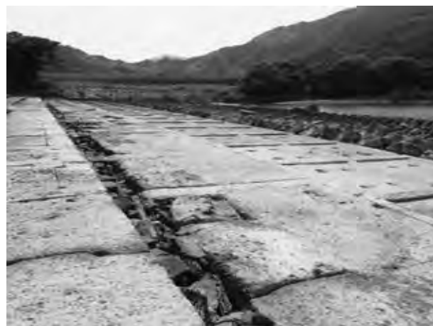
写真-2 着工前南岸堰
