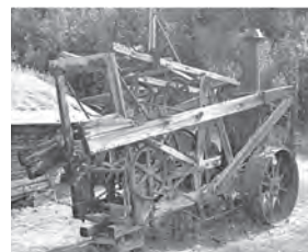
写真一15 Keystone drill
