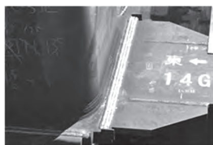
図一3 溶接外観
