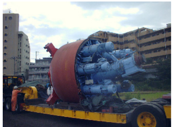
写真-3 掘進機内殻搬入状況
