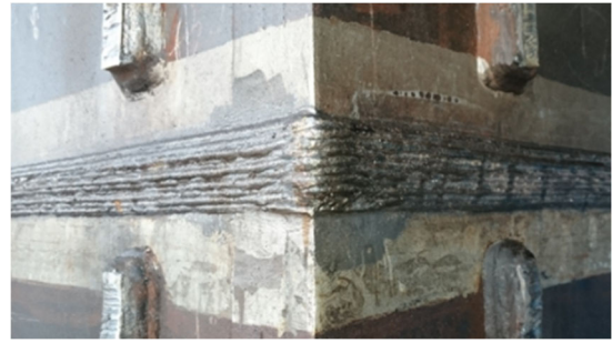
写真-14 溶接外観
