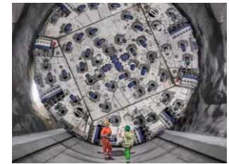
Brenner Base Tunnel
