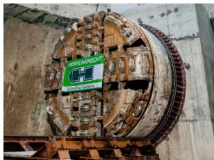
Deep Tunnel Sewerage System
