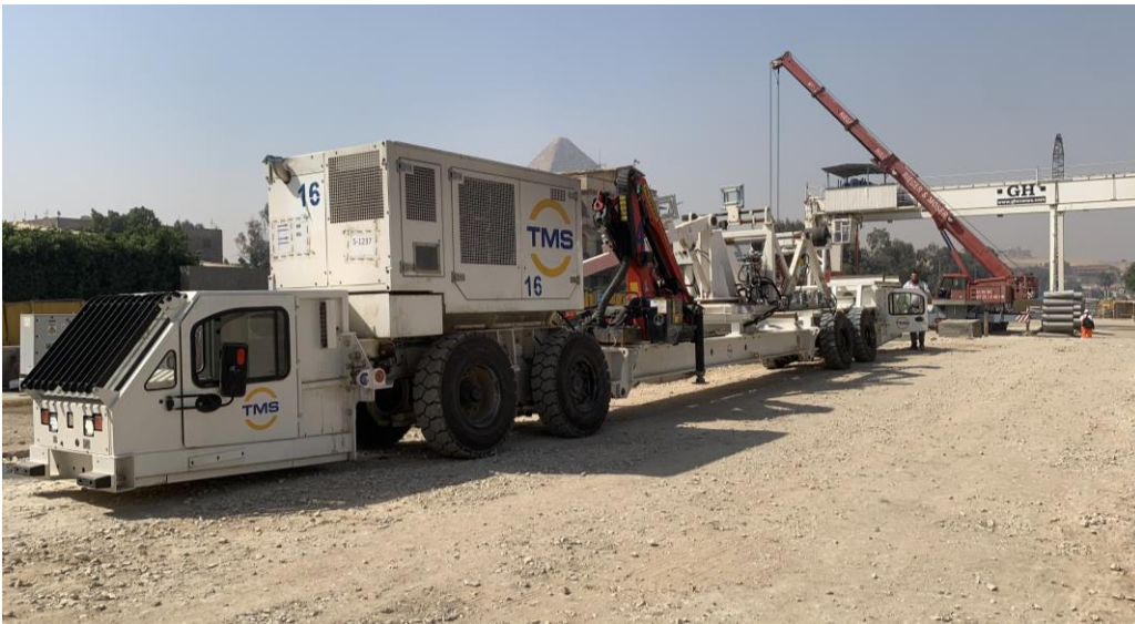
Cairo Metro Line 4 Phase 1 CP401 (Egypt)
