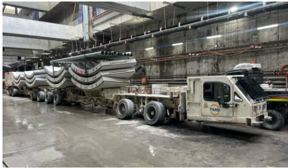
Sydney Metro Western project (Australia)
