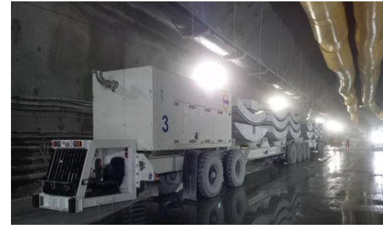
Rishikesh Karnprayag New Rail Line (India)
